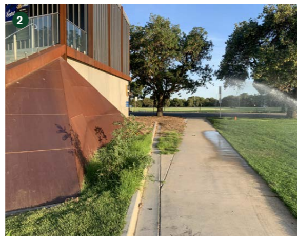
View of garden bed east of Comets building
