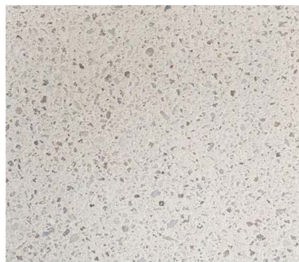
↑ NEW CONCRETE PATH
